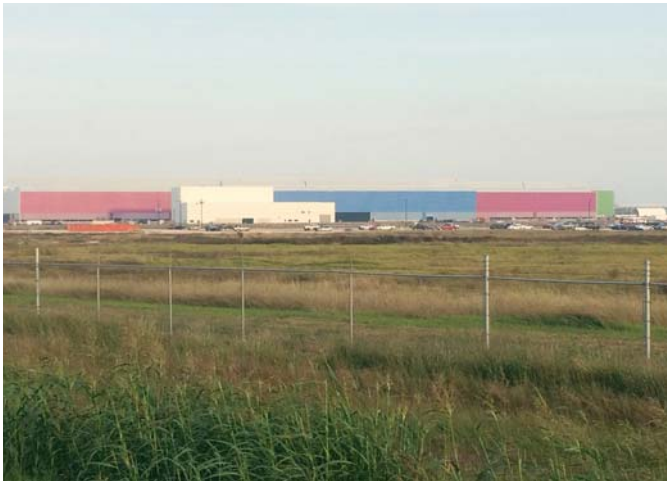
One building of the new Tenaris plant, currently under construction on a former Milberger turfgrass farm, will have 35 acres under one roof.
